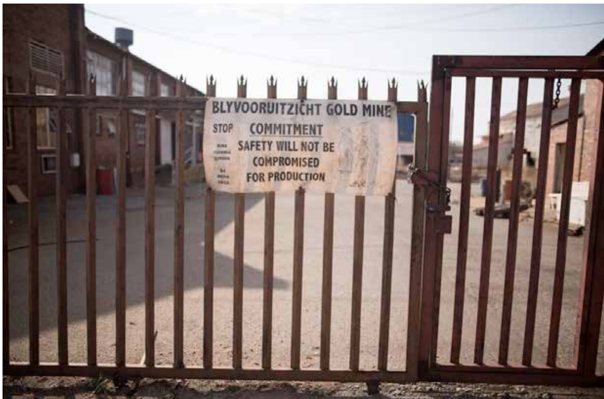
Abandoned Blyvooruitzicht Gold Mine building.
